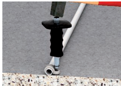
Hammer-in by using setting tool
