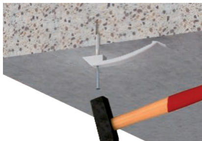
Hammer-in the ceiling
